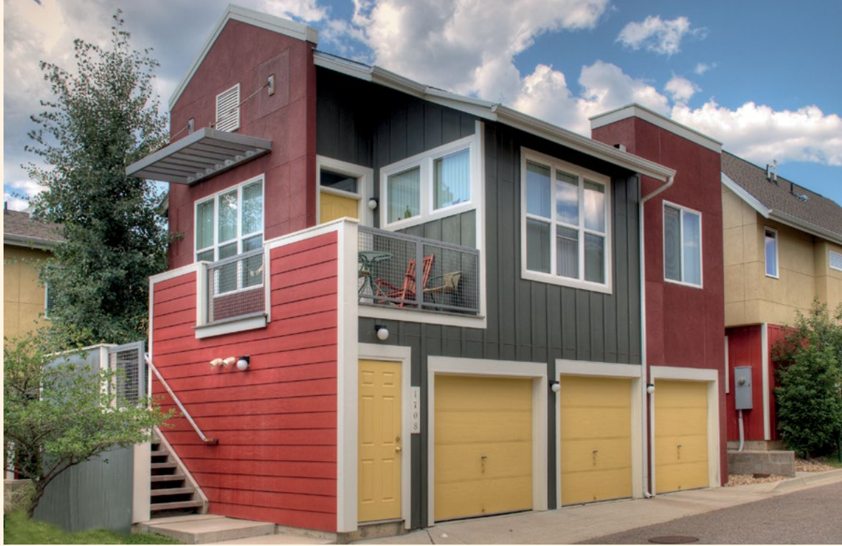
This carriage house ADU, in the mixed-use Holiday neighborhood, is part of Boulder Housing Partners' affordable rental program. Credit: Boulder Housing Partners.
