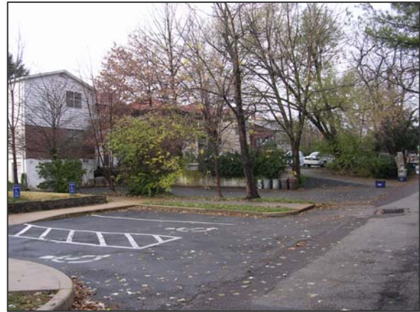
Figure 4—Typical view of CR-UDD from alley looking southwest.
