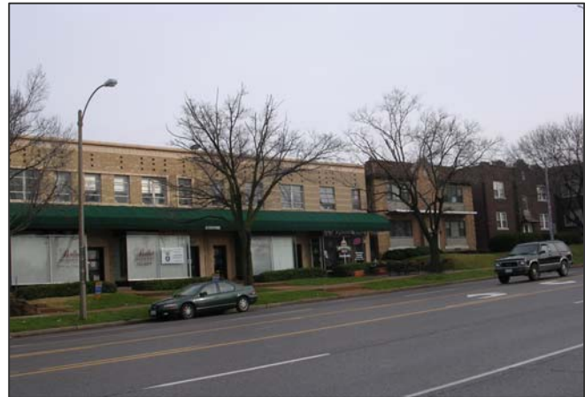
Figure 2—Typical character of original residential and retail storefronts.
